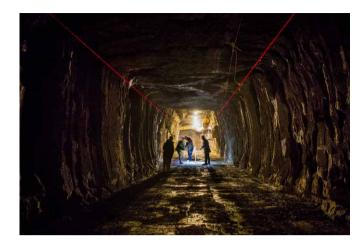
The permafrost tunnel near Fairbanks, Alaska, was built by the United States Army Corps of Engineers in the 1960s and is now used to research and study permafrost. The 110-metre-long tunnel walls contain soil, fossils, frozen animal and plant remains, silt, sand, gravel, bedrock, and thousands of years of history.
