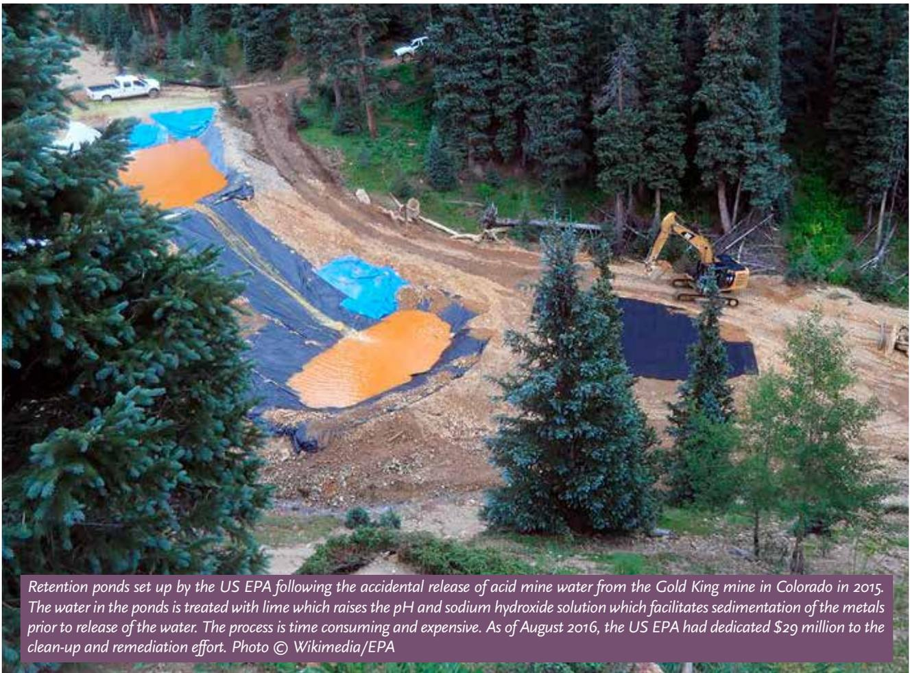
*Retention ponds set up by the US EPA following the accidental release of acid mine water from the Gold King mine in Colorado in 2015. The water in the ponds is treated with lime which raises the pH and sodium hydroxide solution which facilitates sedimentation of the metals prior to release of the water. The process is time consuming and expensive. As of August 2016, the US EPA had dedicated \$29 million to the clean-up and remediation effort. Photo © Wikimedia/EPA*
