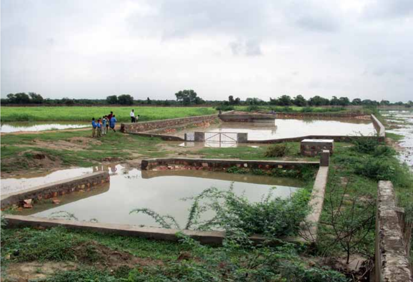
Collection of surface run-off water by the ponds made for groundwater recharging (Chak Ramnagar village, Bharatpur). RSNH Photo Library
