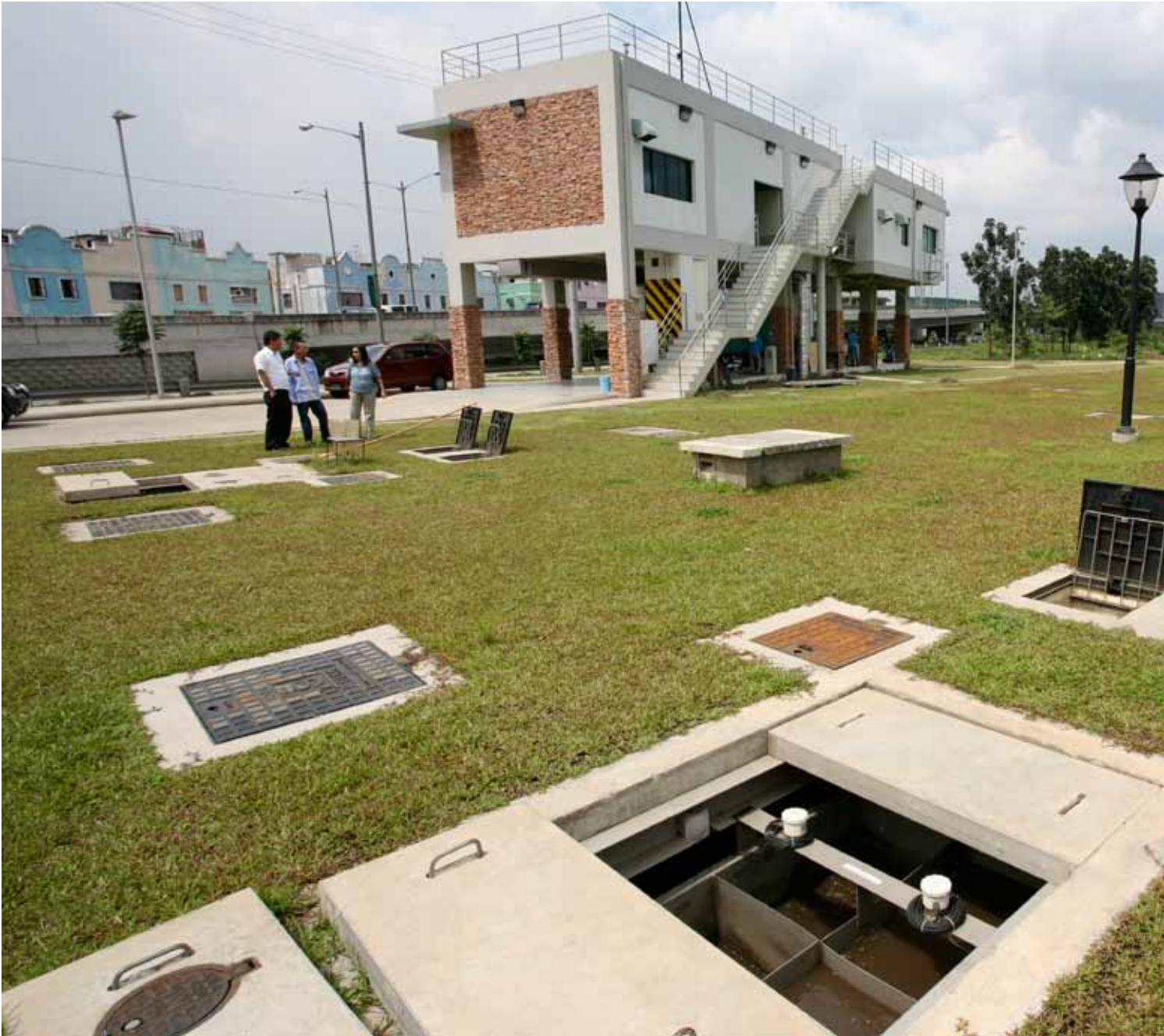
Climate-proofing wastewater treatment facilities is necessary in the face of climate change. Manila Water Company, Inc., one of the two private concessionaires in the Manila metropolitan area, built an elevated facility to counter increased threats from flooding and overflowing rivers. Steve Griffiths
